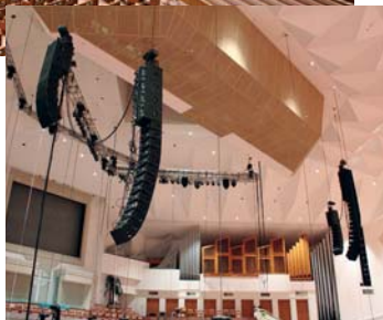
A d&b audiotechnik line array system was selected for its flexibility in dealing with venues ranging in size from 2,000 to 8,000 seats.
